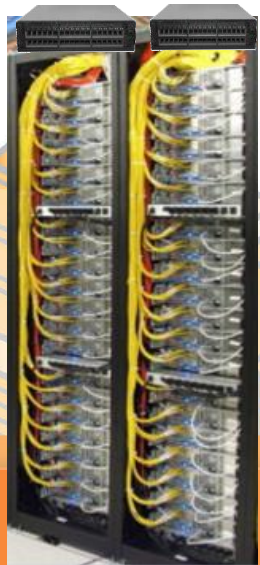
Up & Down the rack Servers & Storage linked to ToR Switches
